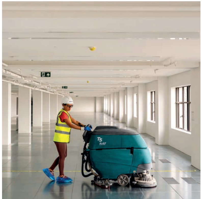
▶ Finishing work on the fit-out of the upper floors
