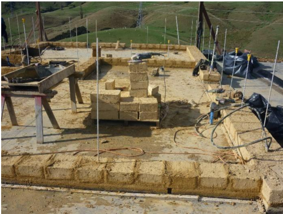
Figure 2: A light adobe house at the beginning of construction (Source: EBANZ )
