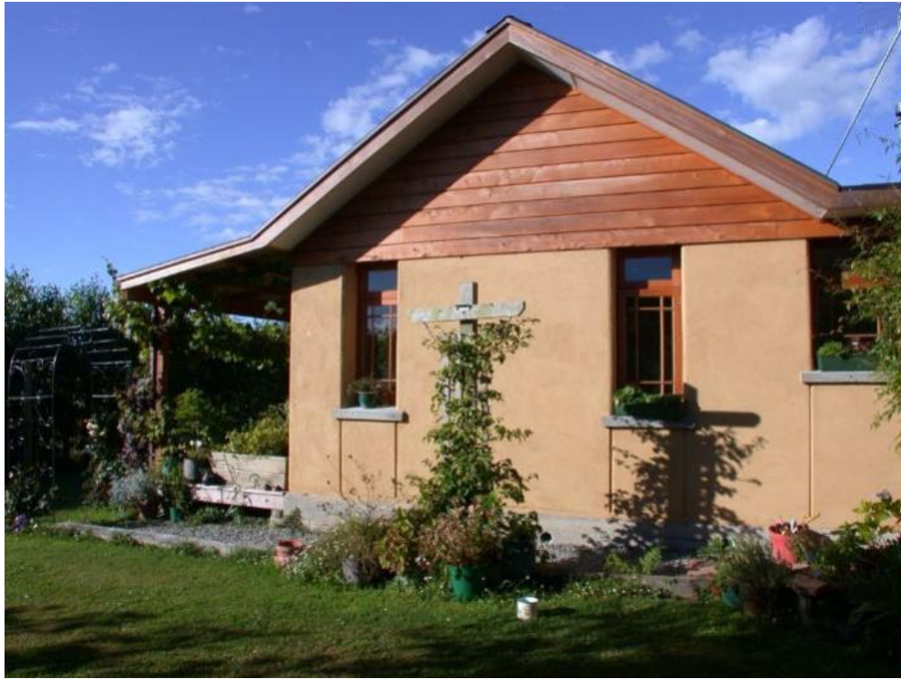
Figure 1: Rammed earth home on the Kapiti (Source: EBANZ )
