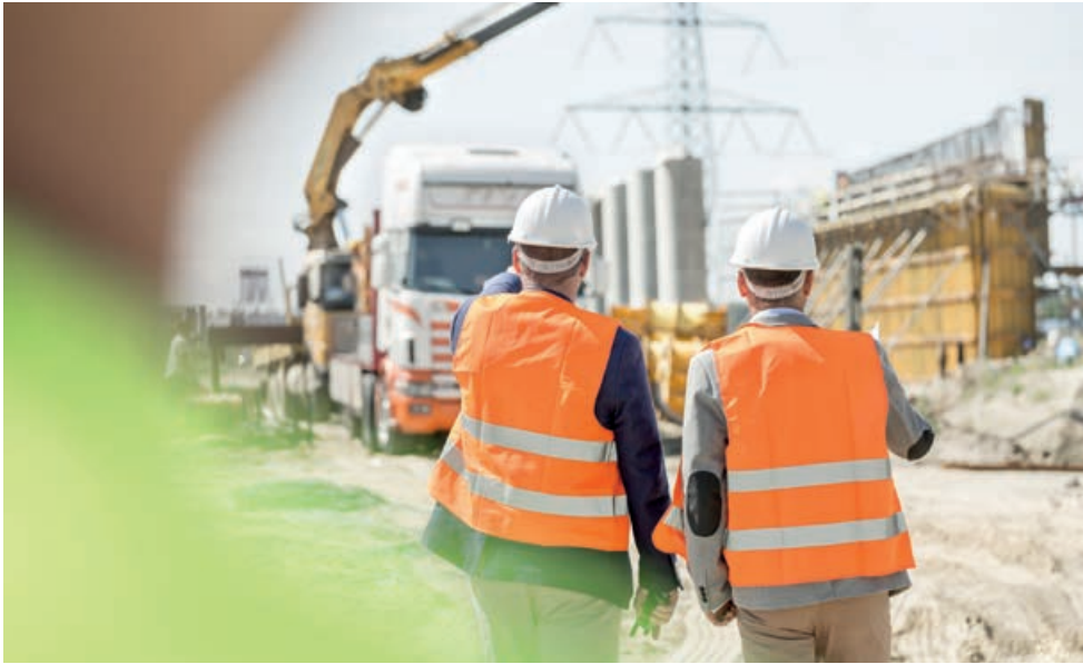
◀ The building control recruitment crisis is complex
