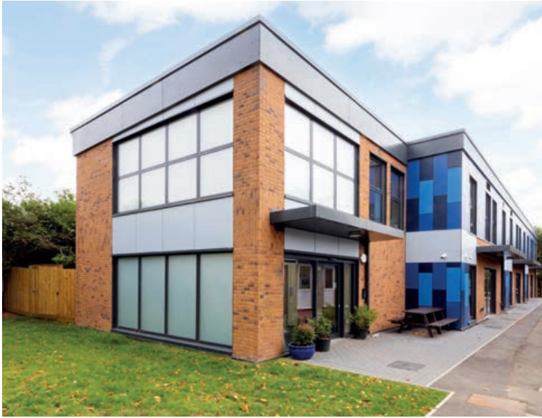
◀ Orchard Hill College Academy Trust appointed Wernick to deliver a two-storey vocational building in St Philip's School in Chessington, Surrey, which was constructed from 22 modules
