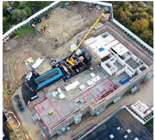
▲ Drone shot of construction progress showing the closed-panel composite timber frame system
