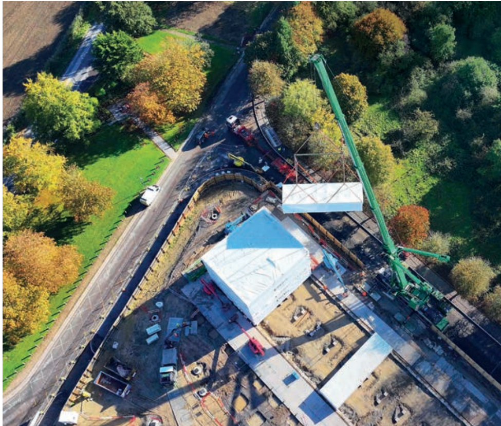
▲ Installation of Merit's pods on site at Moderna, Harwell Campus, Oxfordshire
