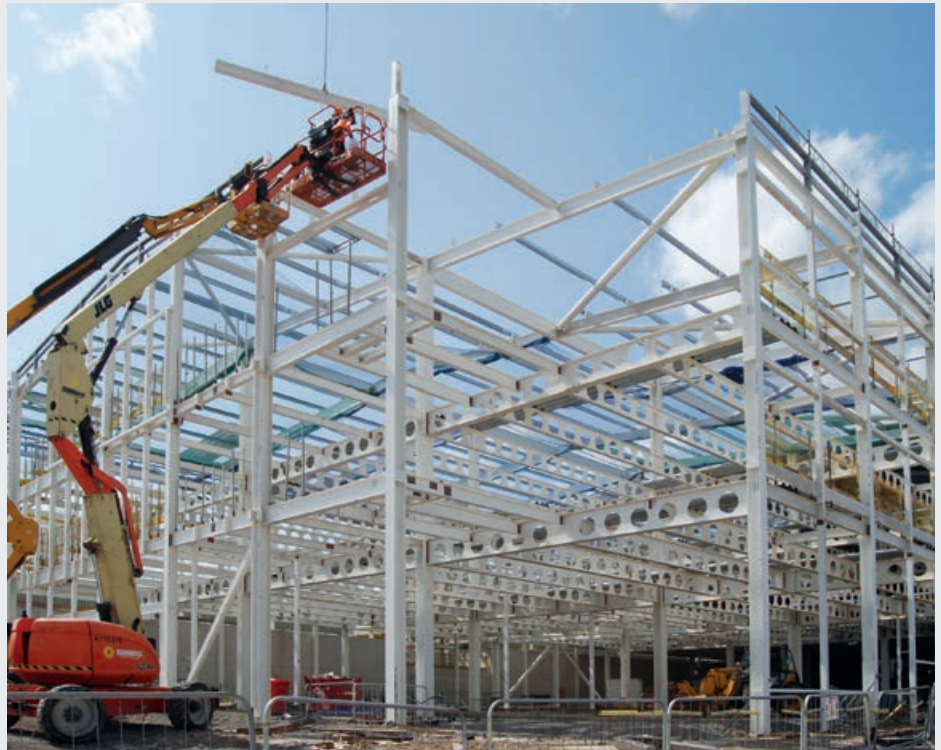
▲ Most of the steel beams are cellular to accommodate the building's numerous service runs
