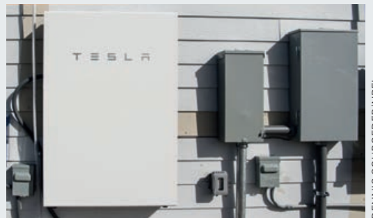
▼ Contractors installed Tesla Powerwall batteries in off-gas homes
