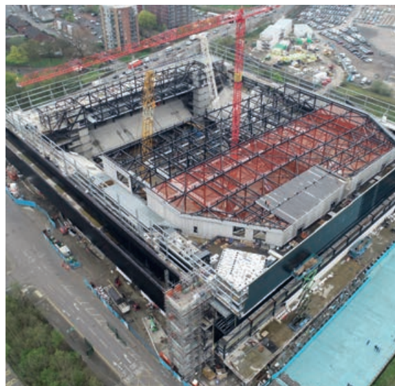
▼ The roof steelwork was erected from inside the building
