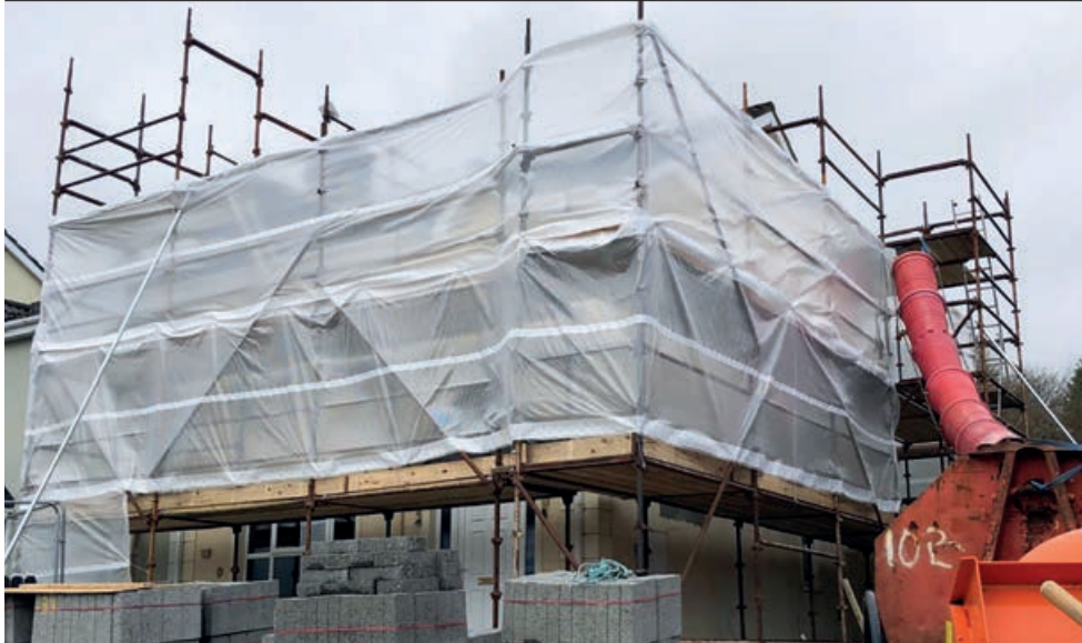
▲ Over the five-month Letterkenny project, the new outer wall was built using 13N concrete blocks, tested for pyrite and mica
