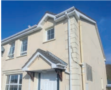
◀ This affected house in Letterkenny, Donegal, needed only its outer block wall replaced. Remediation specialist Anamore used the project to help people understand the remediation process
