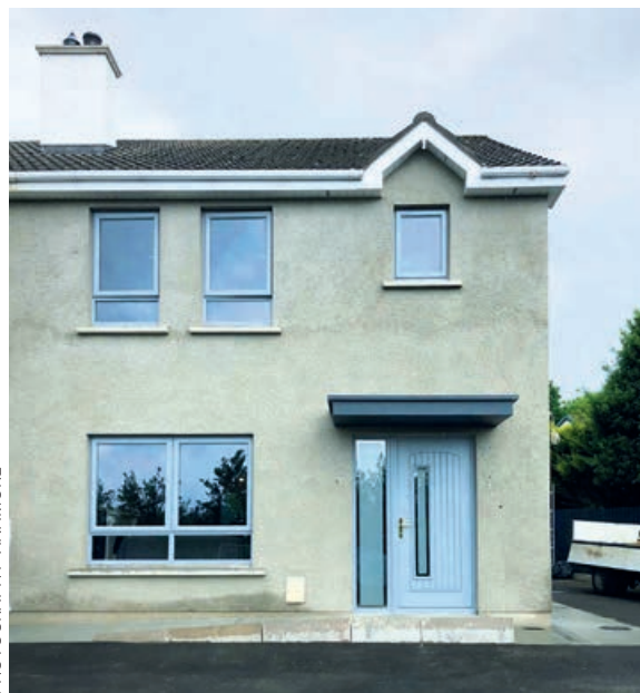
▲ Remediation complete in Letterkenny. Anamore insists on two scratch coats, and strongly recommends a wet pebble dash as the finish because it's more impermeable
