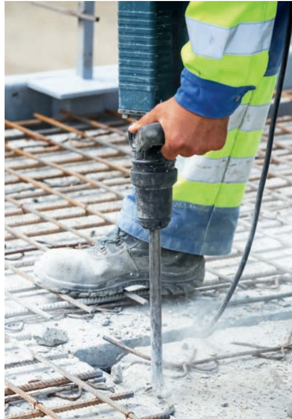
▲ Vibration from handheld power tools can cause damage to nerves, muscles and joints
