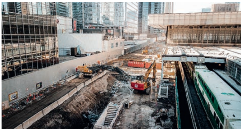
▼ Demolition as Toronto's Union station is expanded
