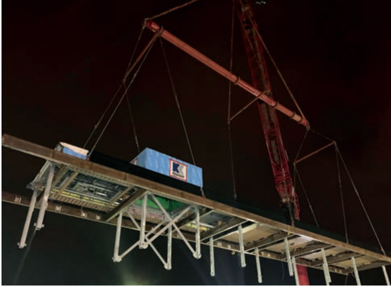
◀ Kenaidan cranes a canopy into place at night
