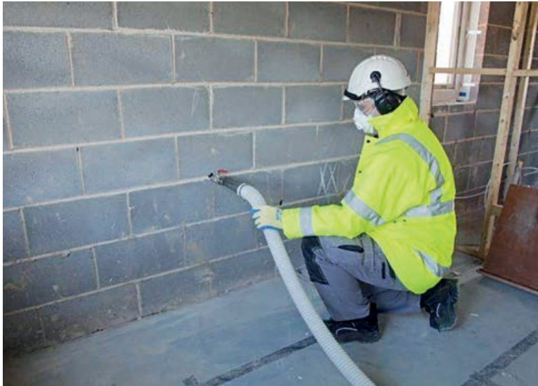
◀ Knauf insulation is applied on a housebuilding project
