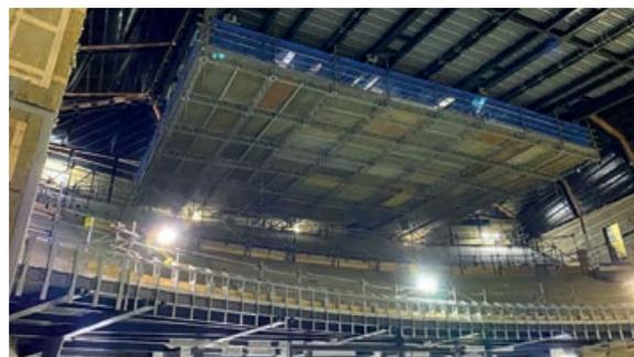
adjacent to the existing platform and then swung out and rotated into position and locked off before being decked out and guardrails fitted.
