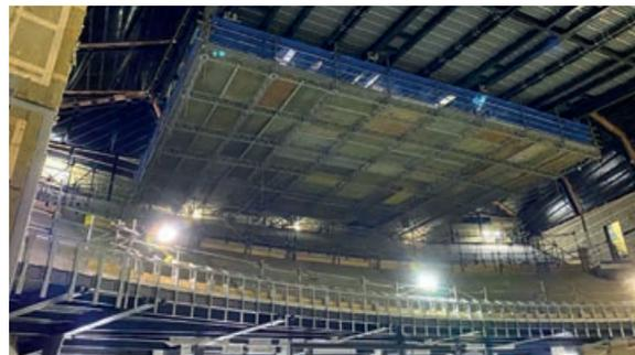
**StepUp Scaffolding UK's GuardAid** Tool, a scaffold positioning tool, enables scaffold configurations to be erected without the risk of fall from height. The erection process ensures that the permanent guardrail is fitted before the platform is installed, and before the scaffolder ascends to the next working lift. The use of GuardAid Tool also ensures the scaffold structure is automatically braced.
