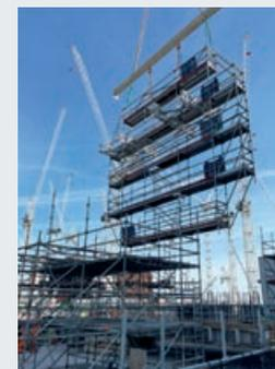
▲ Above: Big Carl, the world's largest crane was needed to lift the suspended scaffold
