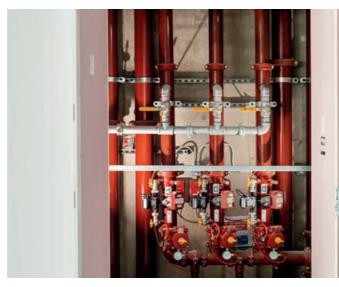
Above: Bi-directionally fire-tested riser doors with adjustable frames installed at 8 Bishopsgate, London
