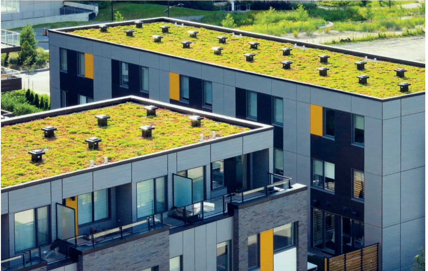
▲ Green roofs must be designed to keep vegetation above any standing water
