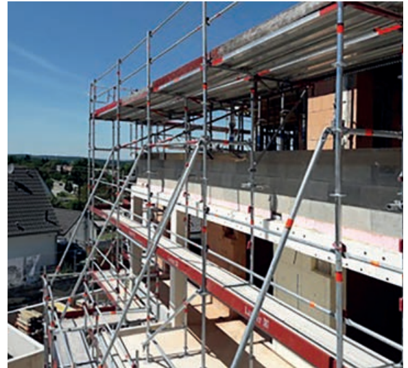
▲ Red levers enable a rapid visual check
