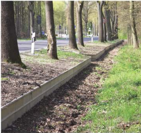
▲ A guide wall is built into the roadside verge to direct animals to the safest places
