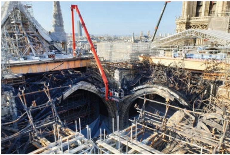
The MEWPs were able to reach down into the centre of the damaged scaffolding
