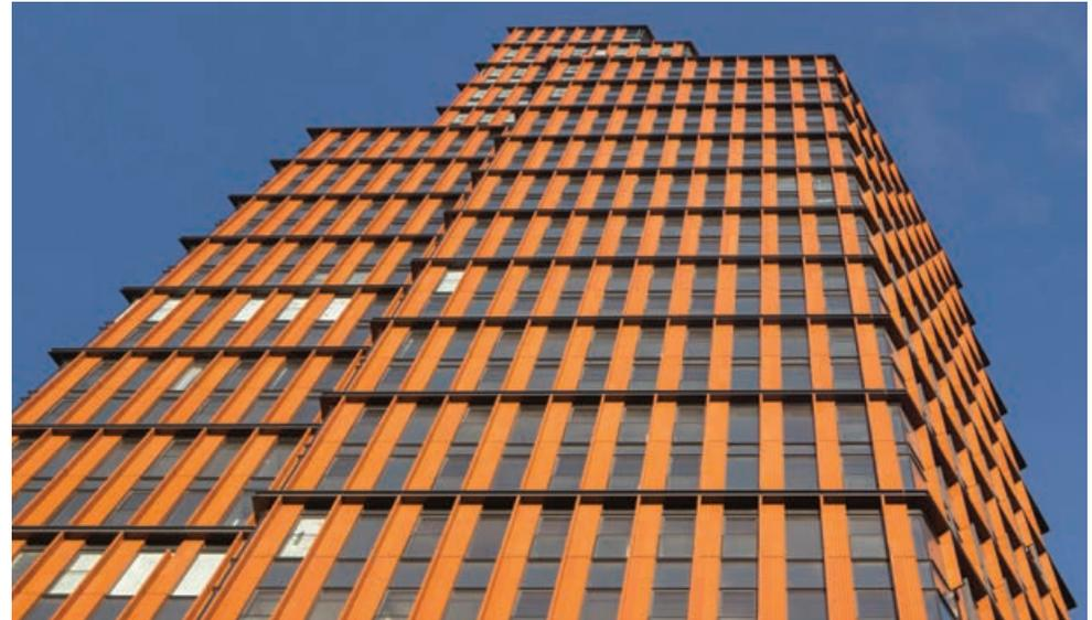
The cladding features glazed terracotta fins on the external perimeters of the towers
