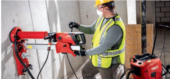
Diamond coring is an alternative method to traditional breaking
