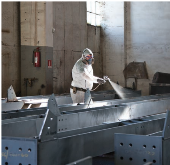
Factory application of intumescent paint
