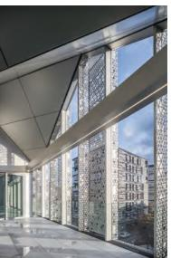
Perforated anodised aluminium panels and glazed curtain walling on the facade
