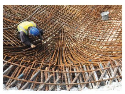
and schedule and another three to four weeks to fix into place. Once it had been installed, the concrete was sprayed on to the moulds.
