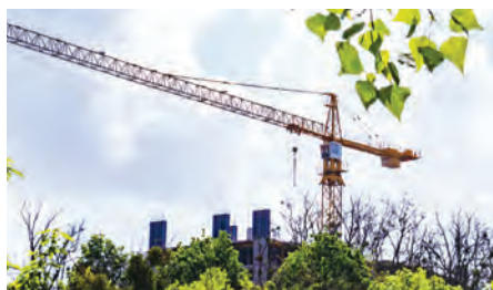
Circular strategies could cut infrastructure emissions by 50%
