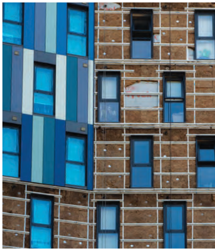
Safety focus: cladding is removed from a student accommodation block in Bristol
