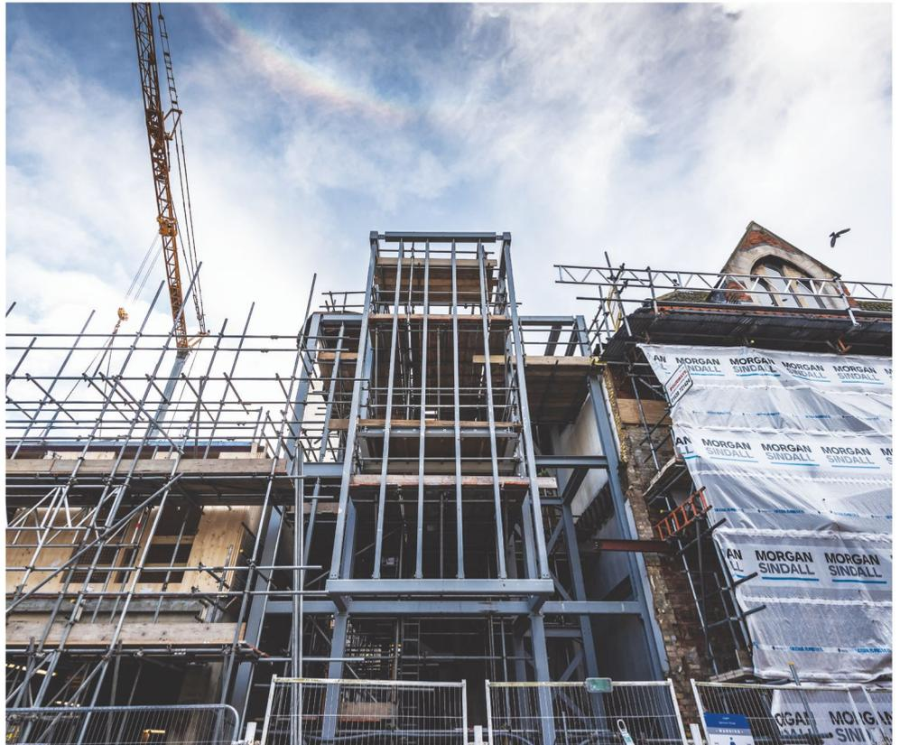
**A steel-framed link building will provide a new entrance and vertical circulation (CGI, top, and during construction, above)**
