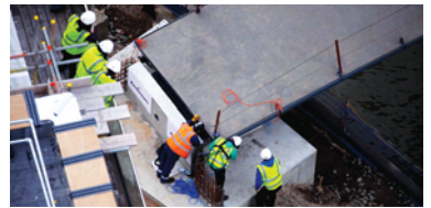
Fixing one of the steel bridges into place
