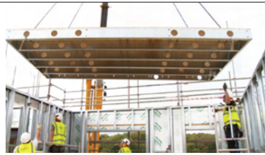
A steel floor cassette is craned into place
