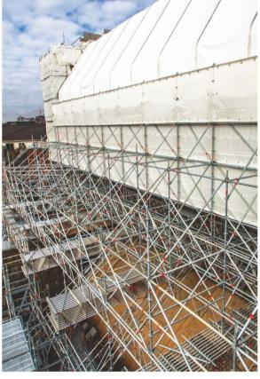
Left: The beam clusters support further structural elements which rise to support the temporary roof Below: The temporary roof spans some 18m
